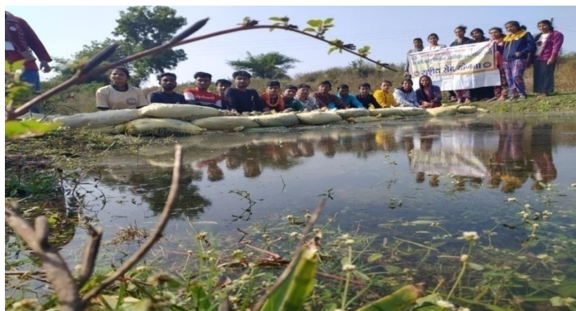
Construction of Gabion Structure by NSS Volunteers at Adopted Village
