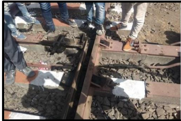
Field Visit at Railway Track gave information about Fuel Feeling Unit
